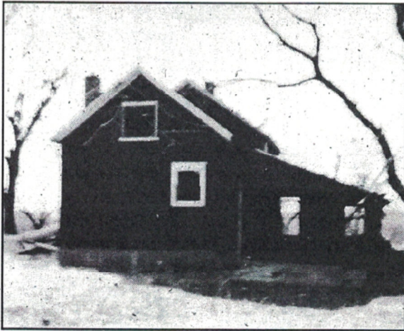
The Caretaker's house on lamprey Hunt Club in 1978 after vandalism.
